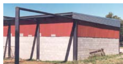
Bunker with pitched sliding roof
