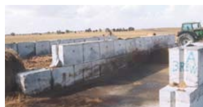
Concrete block bunkers
